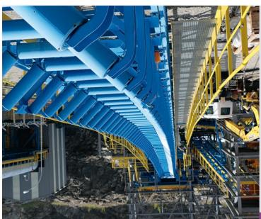
The conveyor belts carry the iron ore 12kms on its way to the ships. The equipment is capable of carrying up to 12 thousand tons of iron ore per hour.
