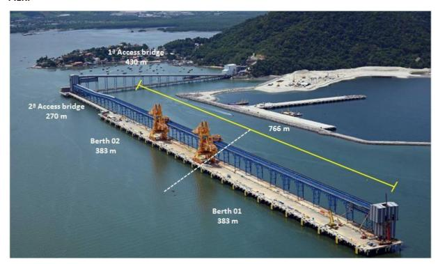
The pier has a total length of 766 meters (two berths) equipped with 27 fenders spaced 28.8 meters from each other.
